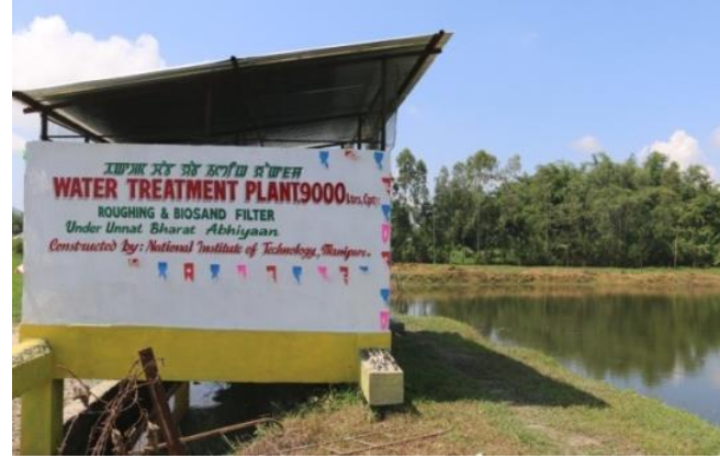
Biosand Filter Water Treatment Plant in NIT Manipur Cluster
